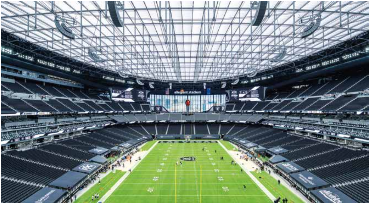
The innovative ETFE roof system provides natural lighting and offers protection from the effects of the weather.
